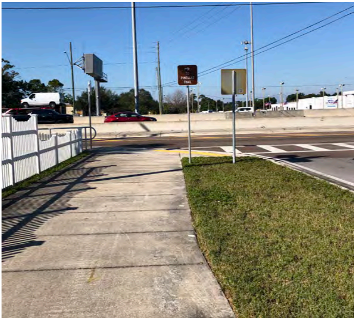
Figure 40. Intersection at Frontage Roads
